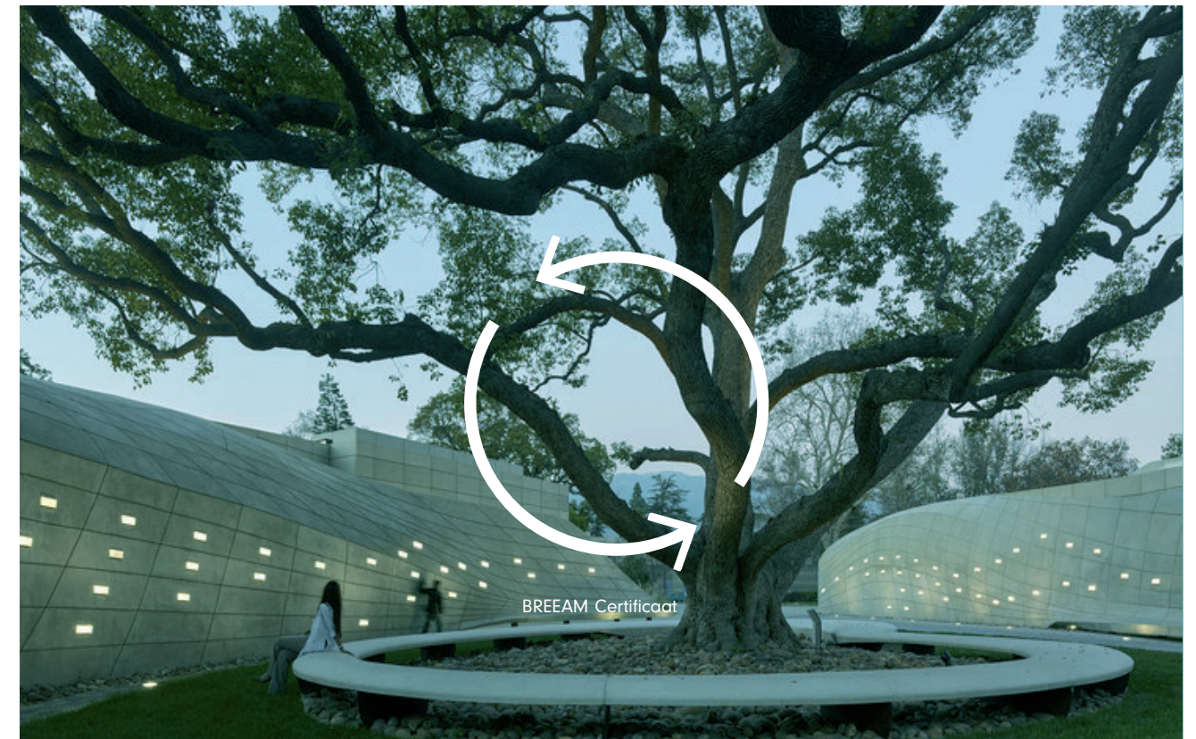
Kaplan Family Pavilion, Belzberg Architects - Duarte
