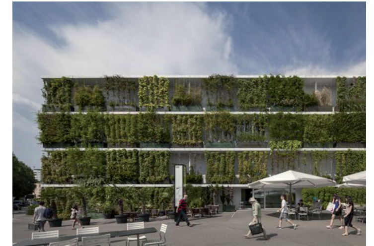
Stucki shopping centre, HRS - Basel
